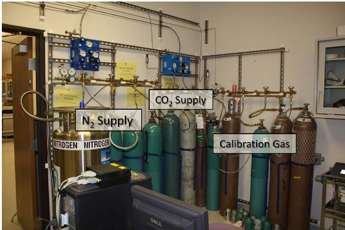
Figure 3-1 MFGCS Gas Supply and Automatic Change Over System. The three subsystems are (left to right): the N_2 supply, the CO_2/N_2 blend supply, and the calibration gas supply.
